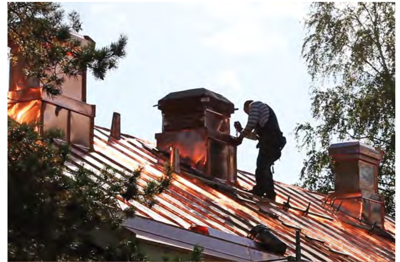
Traditionally, copper has been used as a lightweight, fully supported covering to roofs, walls and other building elements.
